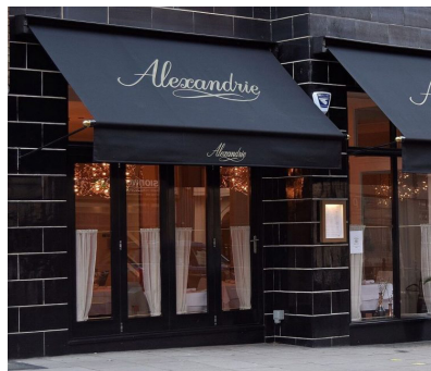
Fig 12. Example awning sign.
