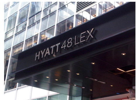
Fig 13. Example canopy sign. Letters may be mounted to the top of the canopy as well.
